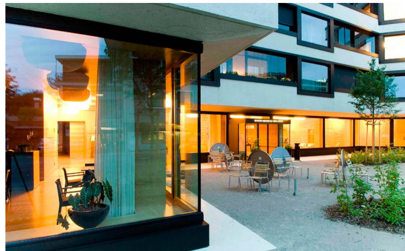
Ground Floor Glazing, Seniorenresidenz Spirgarten
