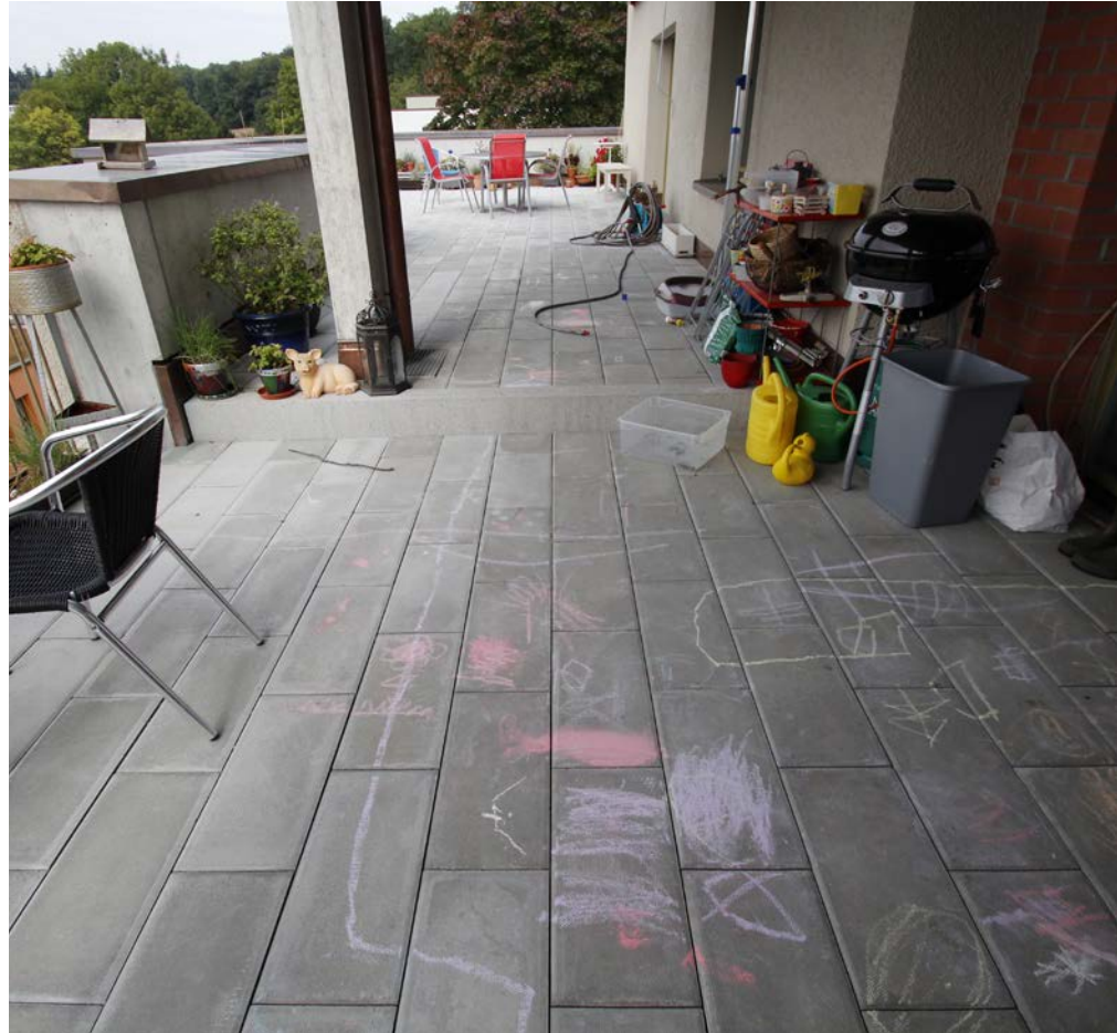
Patio and Stair Landings, Kraftwerk II
