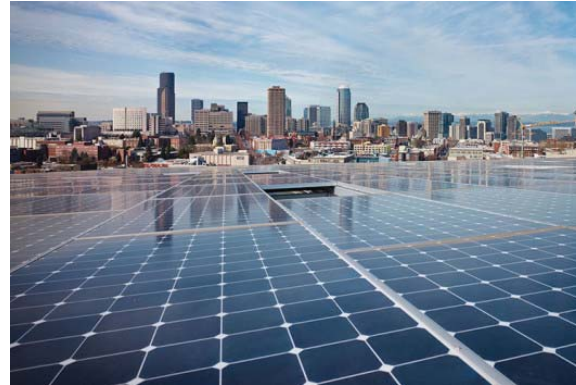
The array of solar panels that is the roof of the Bullitt Center.
