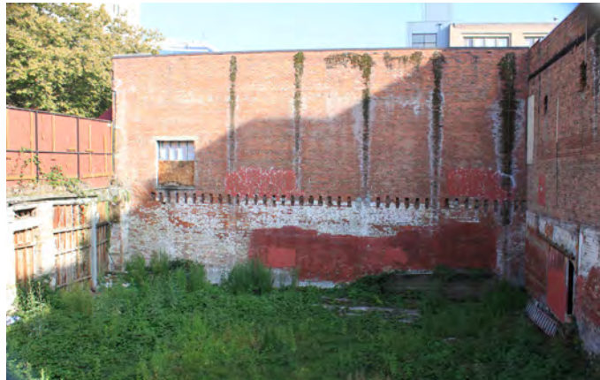
VIEW OF PIT ADJACENT TO NORTHEAST CORNER
