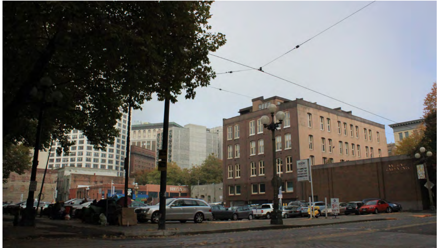
VIEW FROM SOUTHWEST CORNER
