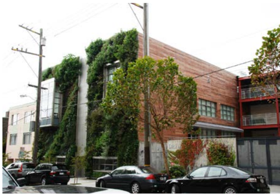
Vertical wall of assembly wing of Drew School
